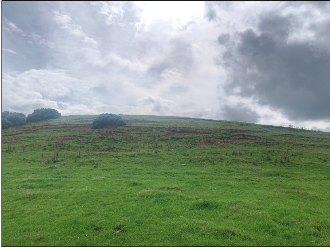
Photo 1: Evidence of soil creep west of T09
